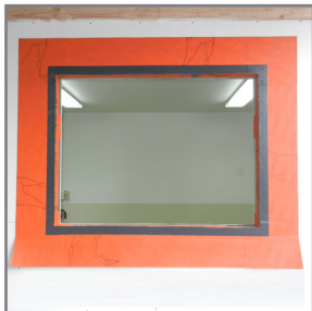
11. Immediately spread the applied material with a putty knife creating a 1" border around the rough opening.
