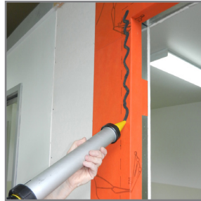
10. Using the sausage gun, apply VaproLiqui-Flash in a zigzag pattern on the wall face surrounding the rough opening.
