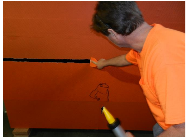
Use a DRY joint knife, trowel, or spatula to tool sealant.
