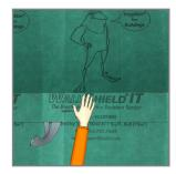
6. Lay overlapping layer of WallShield IT onto vertical sealant joint and smooth with hand pressure.
