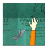
9. Optional for extreme exposure locations: Use the opposite hand to smooth the two layers together as the release film is removed.
