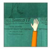
10. Optional for extreme exposure locations: Smooth out wrinkles with hand pressure and seal the adhesive strips using a hand roller.
