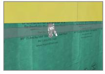
2. Install with SS staples in the top 2" above the Integrated Tape. Avoid stapling in the adhesive strip area of the Integrated Tape.
