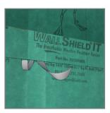
7. Optional for extreme exposure locations: Join horizontal seams by peeling back both release films, starting from where horizontal joint meets vertical joint.
