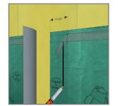
5. Remove release film from top of adhesive strip where flap overlaps.
