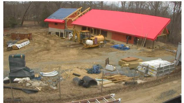
Over 4,600 sq. ft. of SlopeShield SA Self-Adhered Water Resistive Roof Underlayment Sheet (red) was installed on the Alice Ferguson Foundation's Potomac Watershed Study Center. The Potomac Watershed Study Center marks one of several VaproShield projects seeking Living Building Challenge certification. All photos courtesy of TrueLook Webcams.
