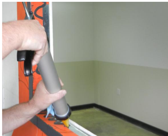
Apply using a profesional caulking gun.
