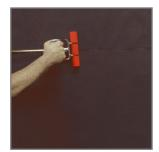
11. Immediately roll the intergrated tape horizontal seams with floor roller to ensure full contact.
