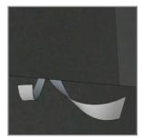
7. Join horizontal seams by peeling back both release films, starting from where horizontal joint meets vertical joint.
